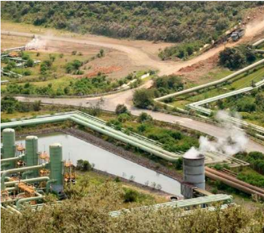
Steam pipes at the geothermal wells in Olkaria KENGEN power stations, Naivasha, Nakuru County on June 2020.
