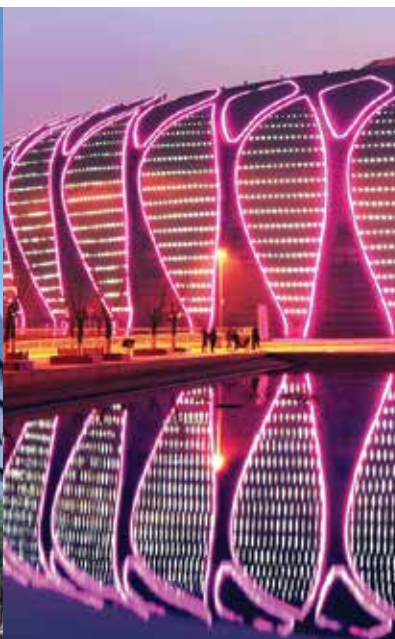
Project: Jinan Olympic Center, Jinan, China Product: Interpon D2015
